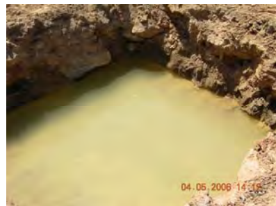
Water Standing in area supposed to be drained by pipe with fabric around it
