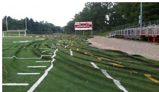
When it is wrong..... rain did this to a field that had a slow draining base
