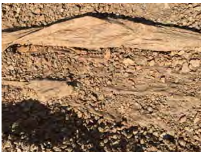
Silted over filter fabric
