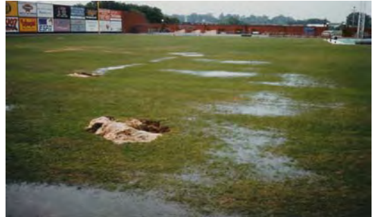
Multiple drain pipes exposed
