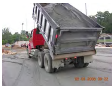
Last load of finish materials backing on field notice no tire rutting
