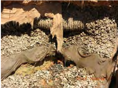
Same area after we cut through the fabric that was silted over
