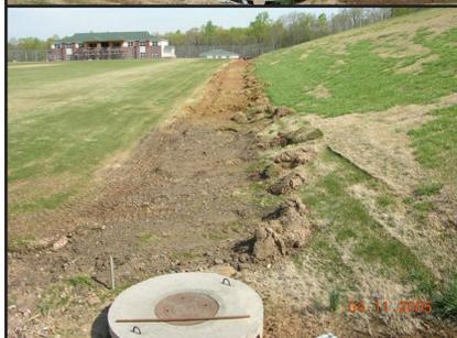
Example of bad conduit installation along edge of a natural turfgrass field and reconstruction to fix it. Photo: Tony L. Strickland, CSFM
