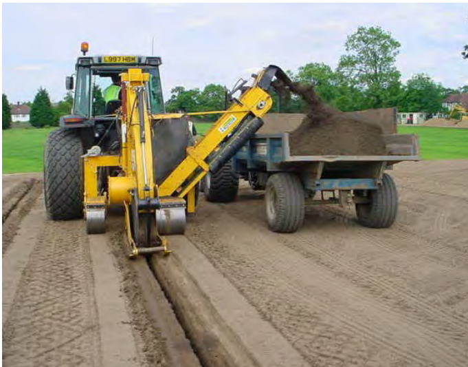
Installation of drainage pipe system - Photo courtesy of Brad Fresenburg, Ph.D.
