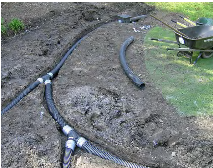
Interceptor drains - Photo courtesy of Brad Fresenburg, Ph.D..
