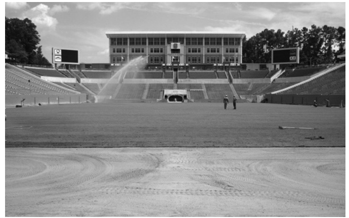
Irrigation of newly installed turfgrass. The use of “big gun” irrigation provides quick coverage and removes heads from the playing surface.
