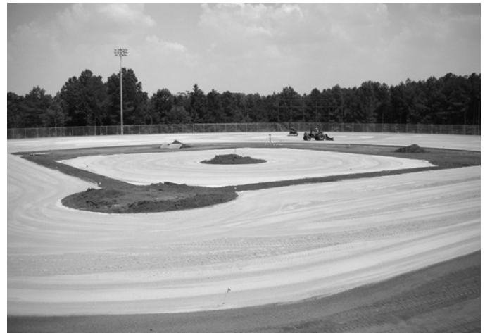
Clay areas of baseball fields require proper grading in relation to the turfgrass surfaces.
