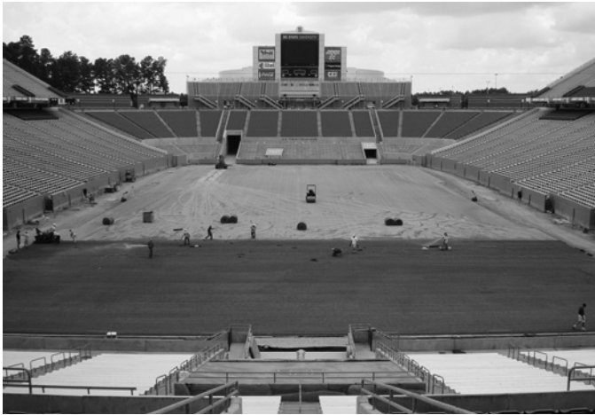
Installation of turfgrass sod on football field.
