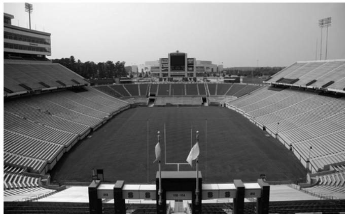
High-capacity football fields are constructed with a sand base to have good internal drainage. Proper construction with drain lines allows for a flatter field.
