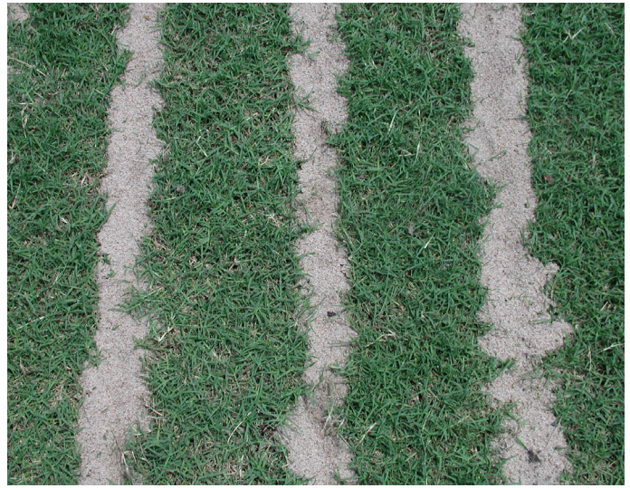
Sand-slit drain trenches backfilled with sand - Photo courtesy of Brad Fresenburg, Ph.D.
