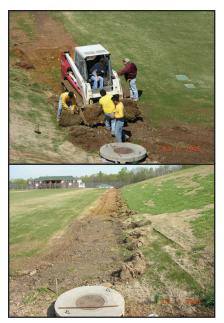
Example of bad conduit installation along edge of a natural turfgrass field and reconstruction to fix it. Photo: Tony L. Strickland, CSFM
