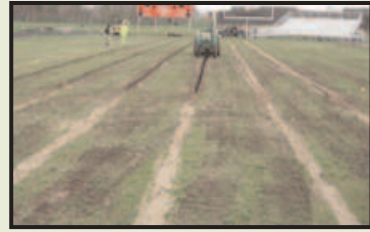
May 2007. Cutting drain lines, installing drain tiles, and backfilling lines with a sand-based root zone material, Grand Blanc High School, Grand Blanc, Mich., Water Management Inc.,
