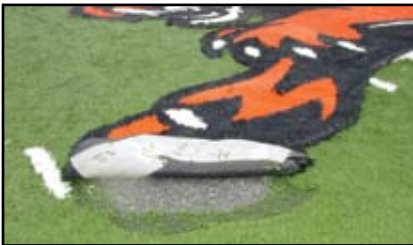
Installation of a special logo on a synthetic field. Photo: Darian Daily
