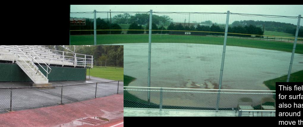
This field has a 1% slope for surface drainage AND it also has French drains around its perimeter to move the water away from the site.
